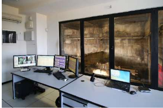
(2) CONTROL SYSTEM AUTOMATIC 24/7
