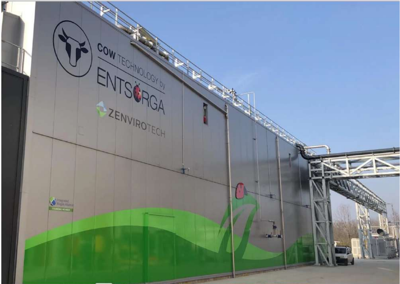
"Cow" anaerobic digester with semi-dry system, developed by EntSORGA in collaboration with Zenvirotech
