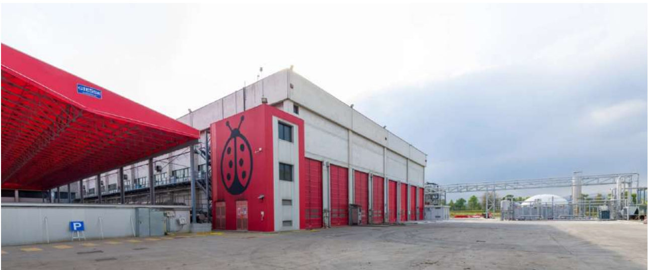
Composting and anaerobic digestion plant in Santhià (VC), designed and built by Entsorga and owned by Territorio e Risorse S.r.l., a 100 percent subsidiary of the IREN Group.
